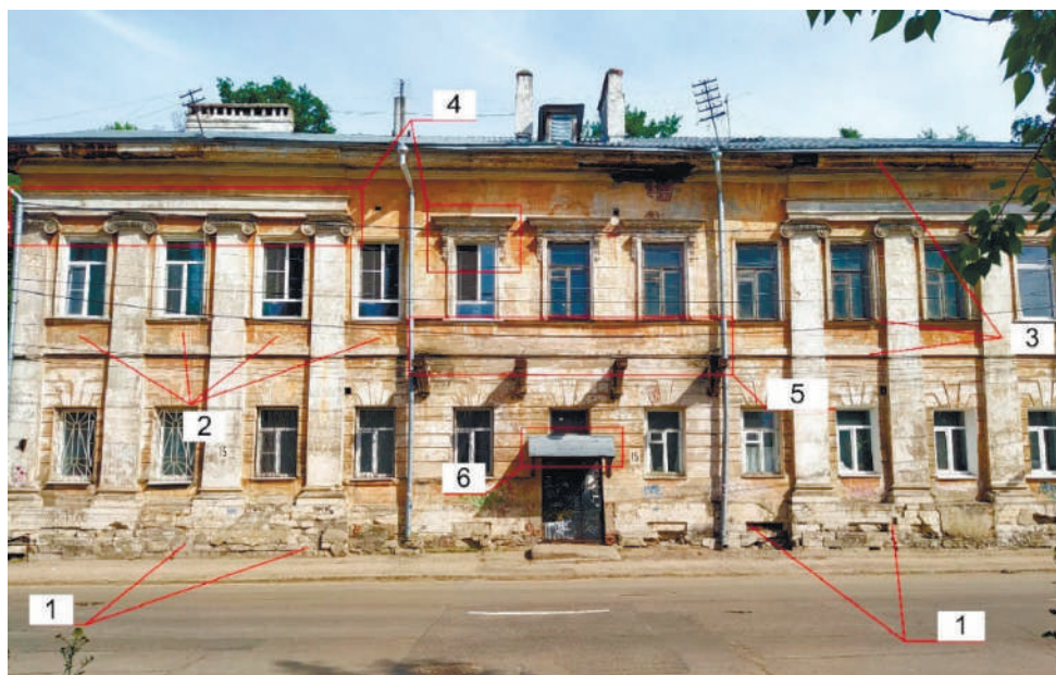
Pic. 6. Restoration of the Nenyukovs' house
