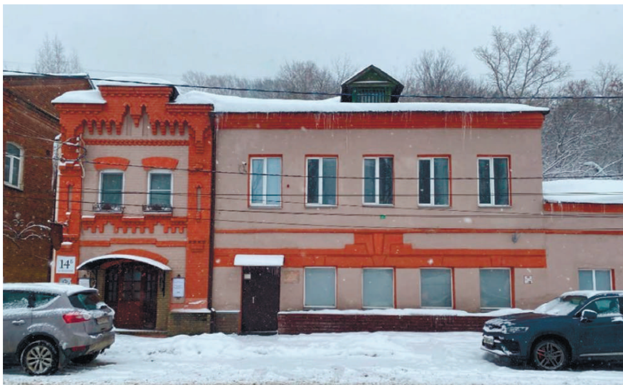
Pic. 3. Chernigovskaya street 14a and 14b
